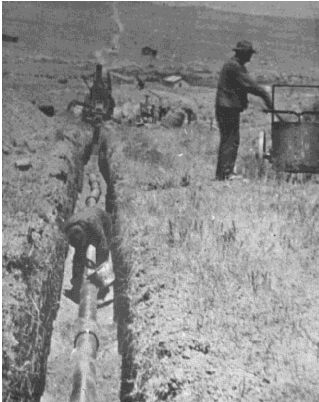
Constructing a pipeline from Salt Creek to Casper, courtesy of Salt Creek Museum, Ed Bille Collection
